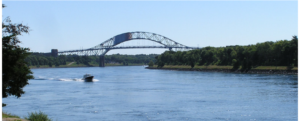
The Cape Cod Canal, looking east toward the Sagamore Bridge with the service road in the foreground, is a beautiful and peaceful sight on a brilliant summer day.
